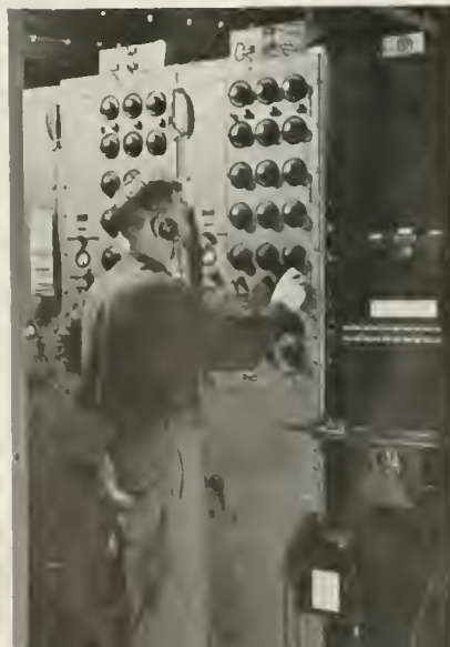
NIEL BECK TUNES A STANDARD RCAC DIVERSITY RECEIVER AT THE NAPLES STATION.
