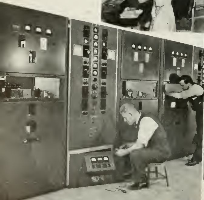
A 5-KW. HIGH FREQUENCY COMMUNICATION TRANSMITTER NEARS COMPLETION.
